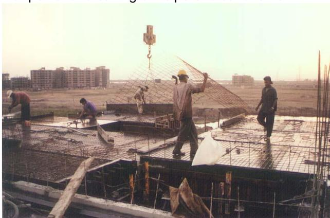
The fabric is available ready to lay on the shuttering. It is also ready for casting as the need for supervisors/ engineers to check the bar sizes & spacings is eliminated. The enormous savings in man-days and the associated cost vary from project to project depending upon the scale of the job and the repeatability of design. Faster execution leading to faster recovery of blocked capital with consequent Interest savings.
