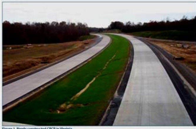
Figure 1. Newly constructed CRCP in Virginia
